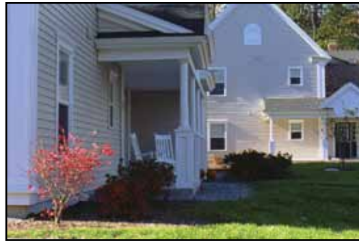
VILLAGE WOODS, YORK | York Housing | Pilot Construction | CWS Architects
